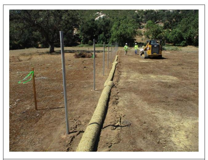
**Photo 6:** Crews were observed installing perimeter chain link fence and fiber rolls at Cuca Loop Staging Yard in accordance with the Erosion Control Plan and SWPPP (MM HYD-1, MM BIO-7).
