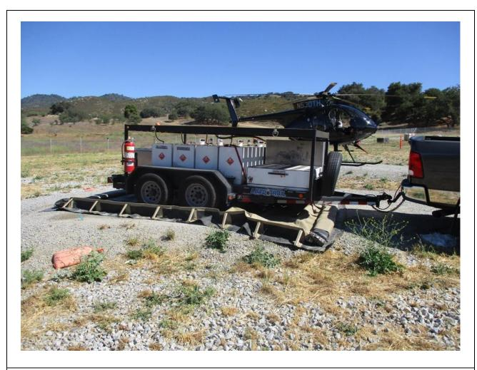
**Photo 5:** To prevent leaks/spills from being discharged into the soil, pop-up secondary containment was observed beneath a fuel tank at Love Valley Yard in accordance with the Spill Response and Notification Plan and MM PHS-2.
