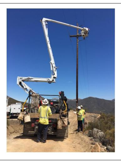
**Photo 2:** Biological monitors were observed monitoring crews during wire spreading activities per MM BIO-22. Insulator brackets were observed being tapped off under the supervision of biological monitors in order to dissuade birds from nesting on the pole and attachments at location Z571462 (TL 6957).
