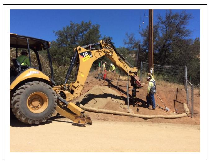
**Photo 4:** During pole and anchor excavation at Pole P870072 (TL6957), all required fire tools (5-gallon backpack pump, round point shovel, Pulaski, and 2A10BC fire extinguisher) were staged on site in accordance with the CFPPP.
